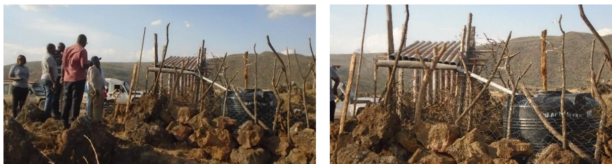
Figure 17: A view of drinking water harvesting at Fumaroles in Suswa project area
