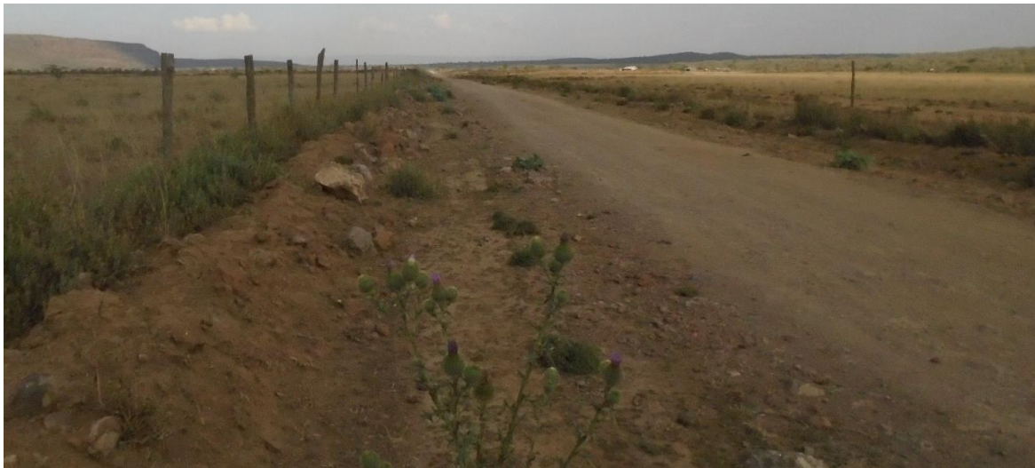
Figure 27: A view of the access road to the site
